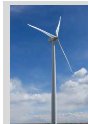
A 1.5-MW wind turbine located at NREL's Flatirons Campus is being prepared for downwind operation. Photo by Jeroen van Dam, NREL
